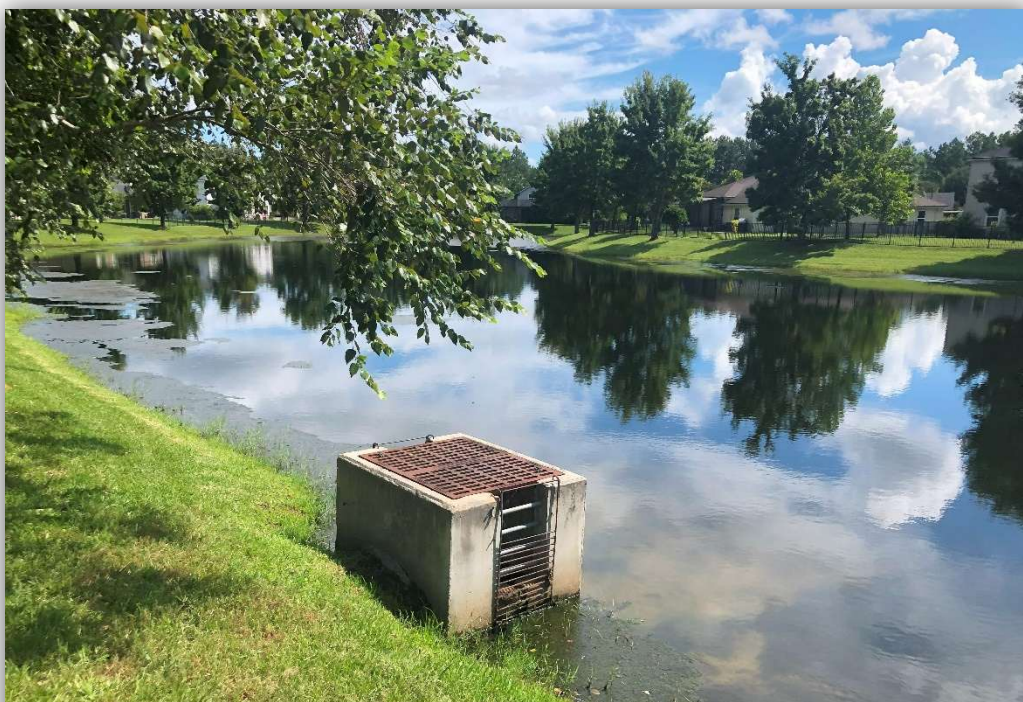
Control Structure at SWMF 3
